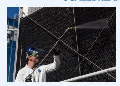
Goodway's ScaleBreak-Gel is a patented, innovative viscous gel formulated for descaling vertical surfaces like cooling tower fill. When used in conjunction with Goodway's TFC-200 system, ScaleBreak-Gel adheres to vertical surfaces allowing its powerful descaling properties to penetrate and dissolve water formed deposits into a liquid suspension for easy removal.
